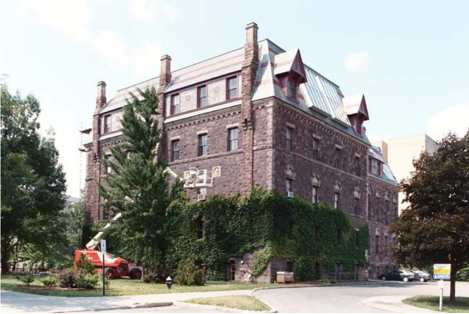
Figure 44 Tjaden Hall, view from northeast
