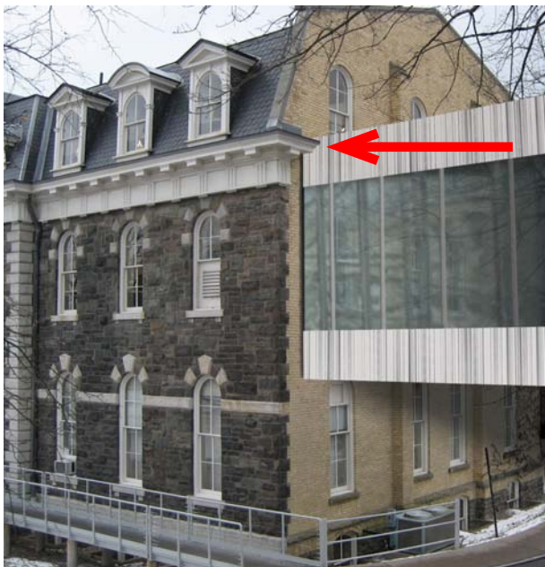
Figure 4.1.25: "Preserved Cornice." Current design scheme for the south facade of Milstein at Sibley's southwest corner. Red arrow indicates preserved cornice.
