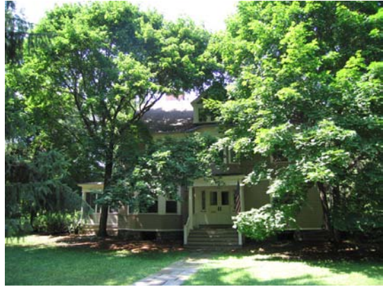
225 Fall Creek Drive (south side)
