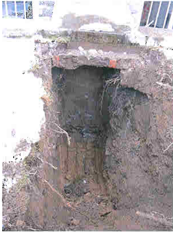
Test Pit –B
