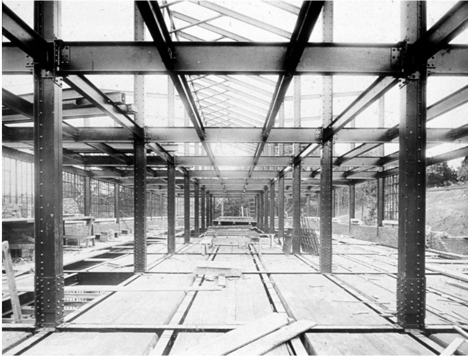
Figure 16 Rand Hall under construction
