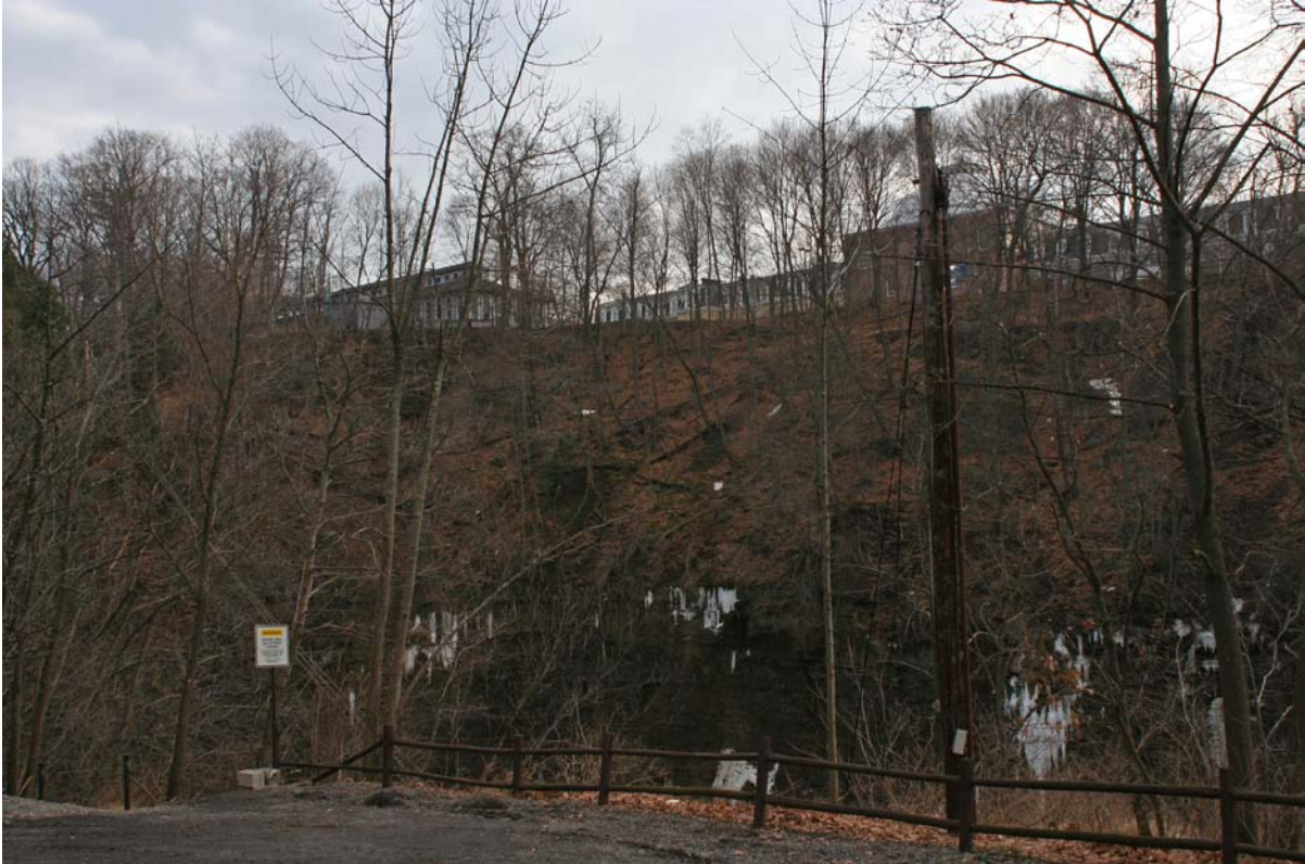
Figure 2.5.34: Existing view from north rim of gorge looking south.
