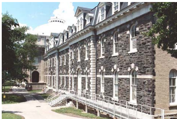
Figure 2.6.2: South stone facade of Sibley trimmed with cut stone, Classical dome beyond.
