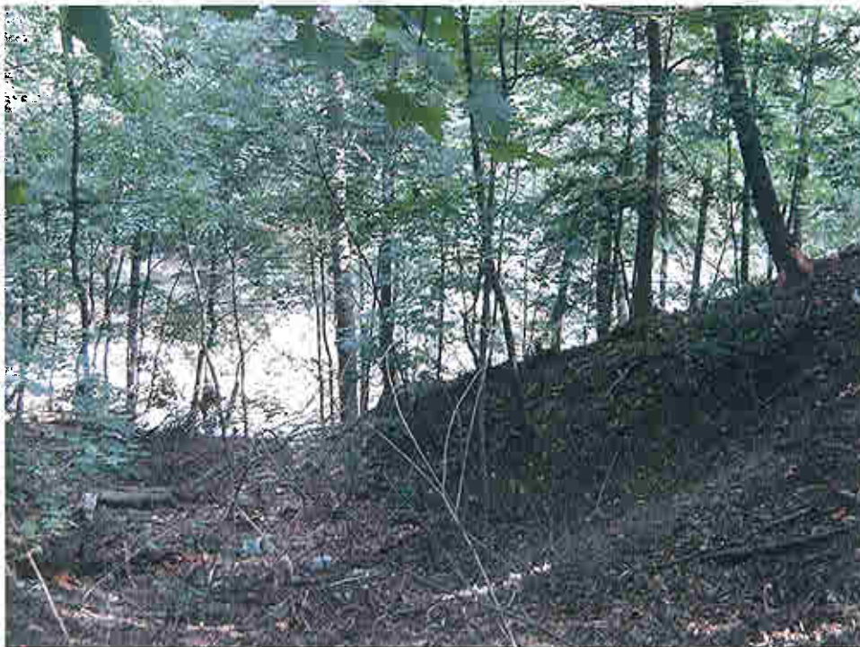
Photo 2 - Area of continuing and historic (1988 ESI Report) large slope failure.
