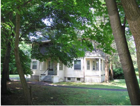
207 Fall Creek Drive (south side)
