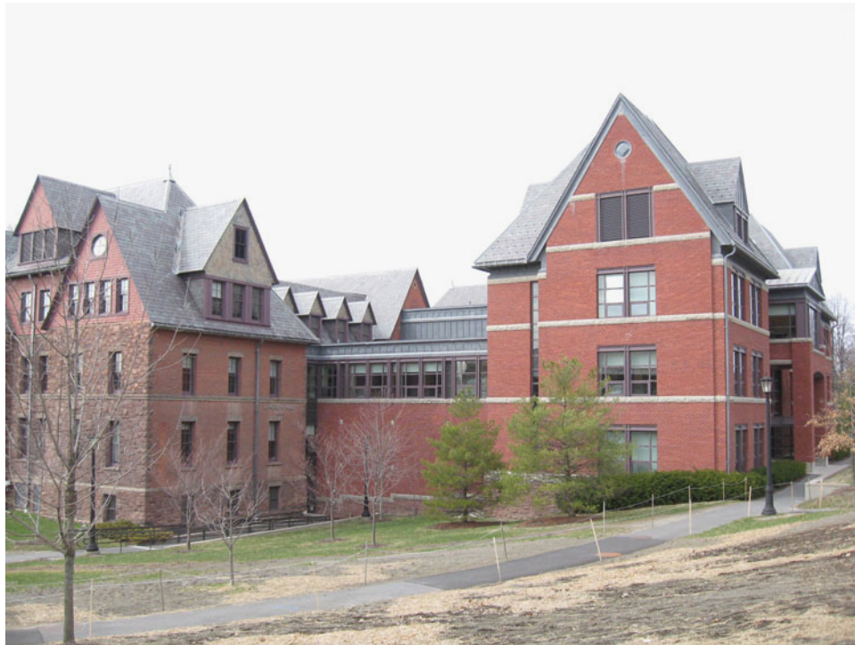
Figure 29. View of Lincoln Hall showing contextual design. The 2000 addition on the right has massing, forms, materials, and details similar to, but not matching, the original building.
