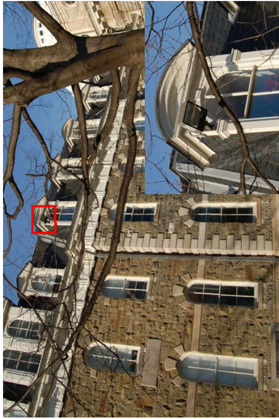
FLOOD LIGHTS MOUNTED TO SIBLEY HALL FLOOD LIGHTING QUAD
