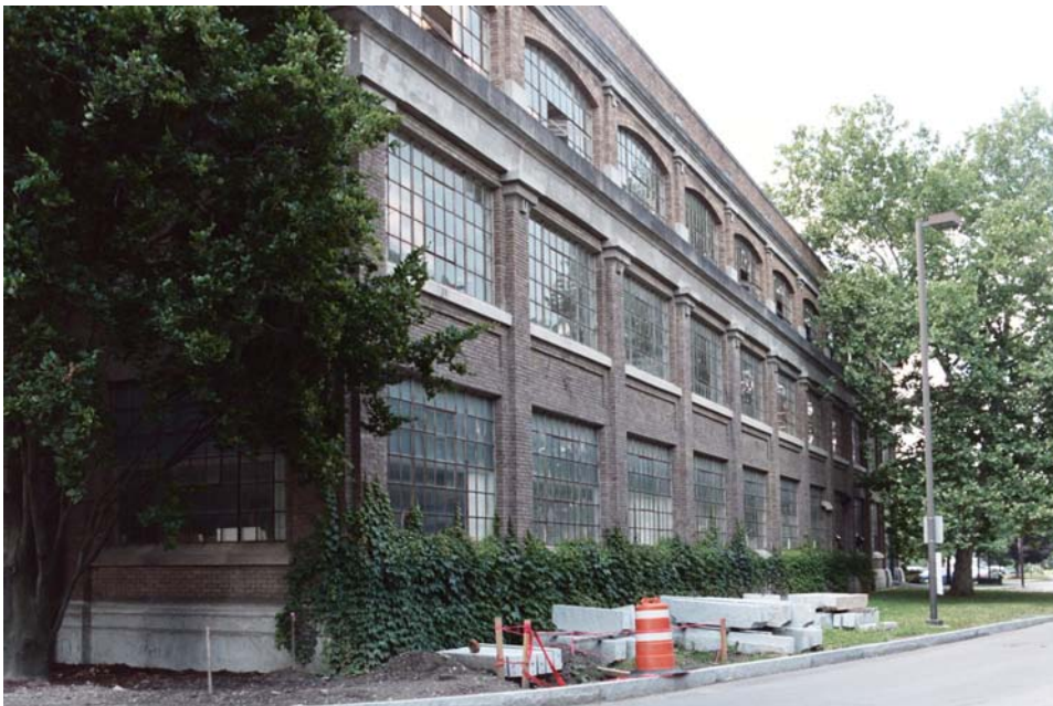
Figure 29 Rand Hall from the northeast
