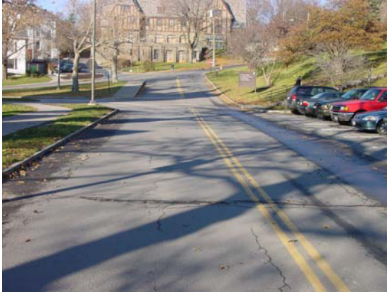
Figure 2.8.5: Looking north along West Avenue toward the University Avenue intersection.
