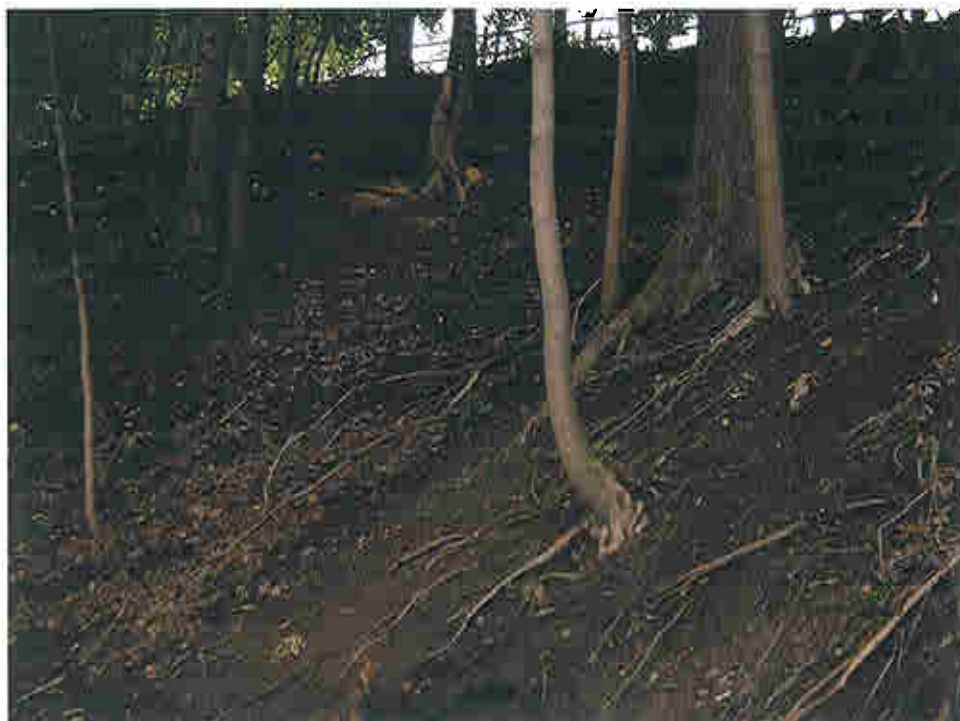
Photo 14 - Looking up to University Avenue from the foot trail, over a barren, eroded area.
