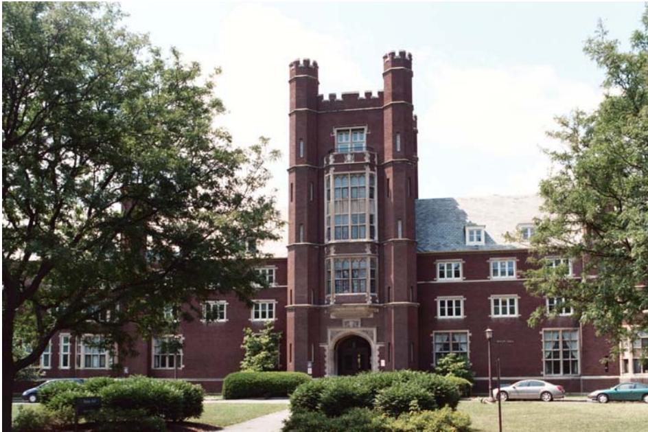
Figure 48 Risley Hall – north façade
