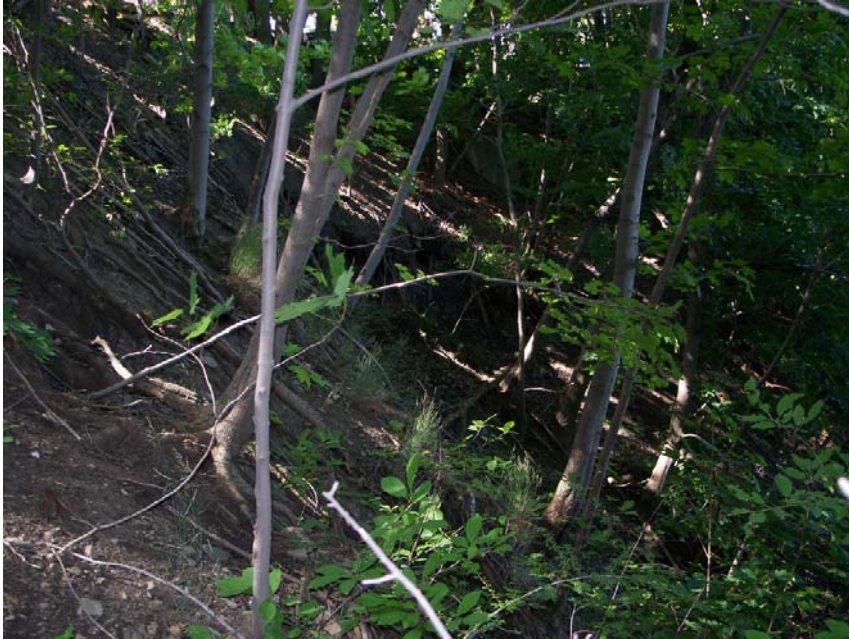
Slope Northwest of Foundry – note exposed roots and large eroded area in center. 07.13.07
