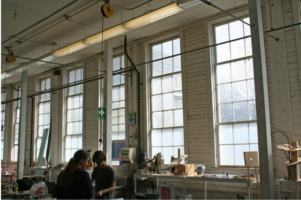
Figure 2.5.28: Existing view from inside the Foundry looking south.
