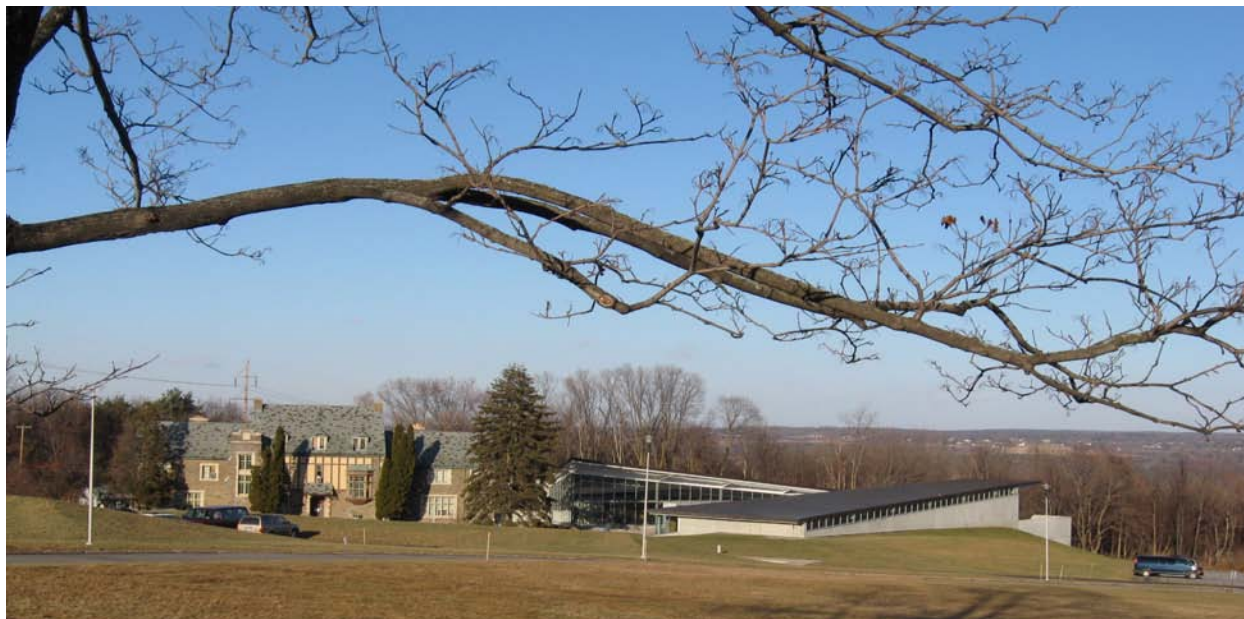
Figure 2.6.5: The Museum of the Earth addition contrasts with the historic Paleontological Research Institution building. The addition, which emphasizes differentiation and removability, is clearly a product of its time. This project was reviewed by the State Office of Parks, Recreation, and Historic Preservation and was found to be in compliance with the Secretary of the Interior's Standards for Rehabilitation.
