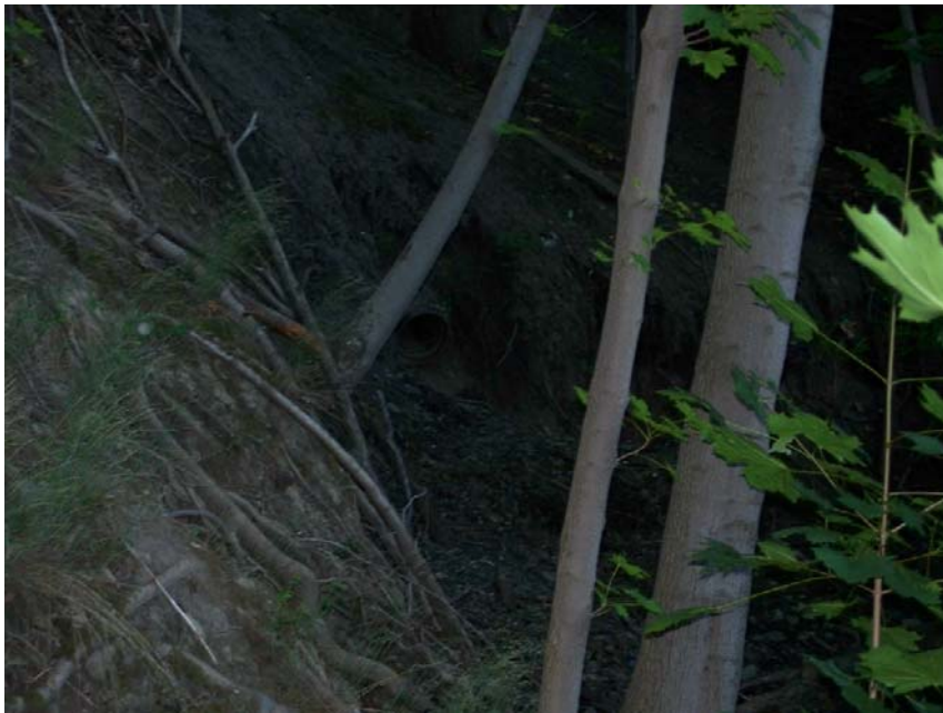
Slope NW of Foundry. Note Drain Tile at center. 07.13.07
