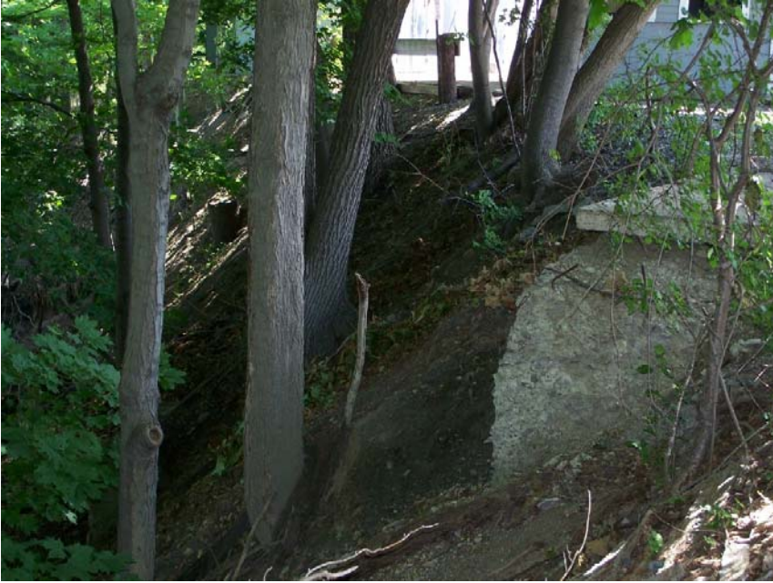
Looking east at concrete fill, slab and slope NW of Foundry. 07.13.07
