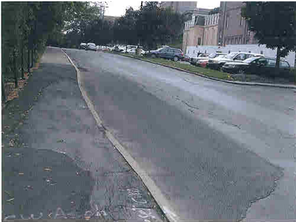
Photo 10 - New asphalt patch (overlay) designated over existing failed area.
