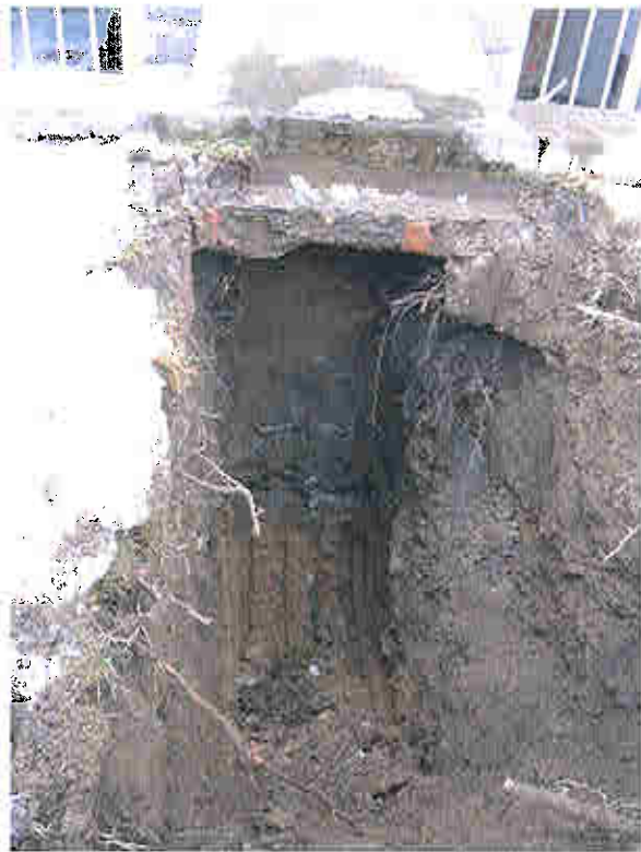
Test Pit –B
