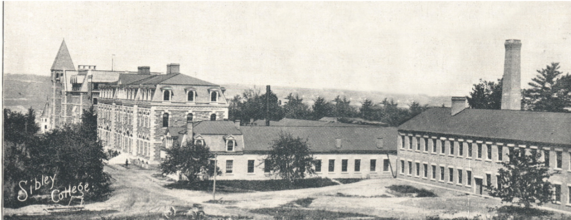
Figure 6. Another view of East Sibley from the east showing some of the workshops
