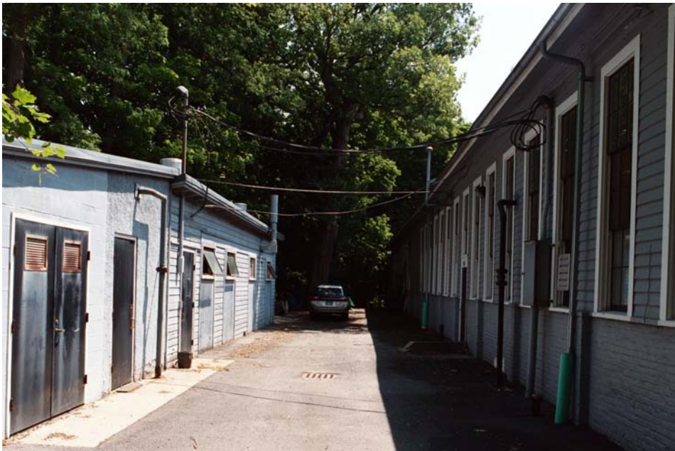
Figure 31 The Foundry, rear façade and shed, looking east
