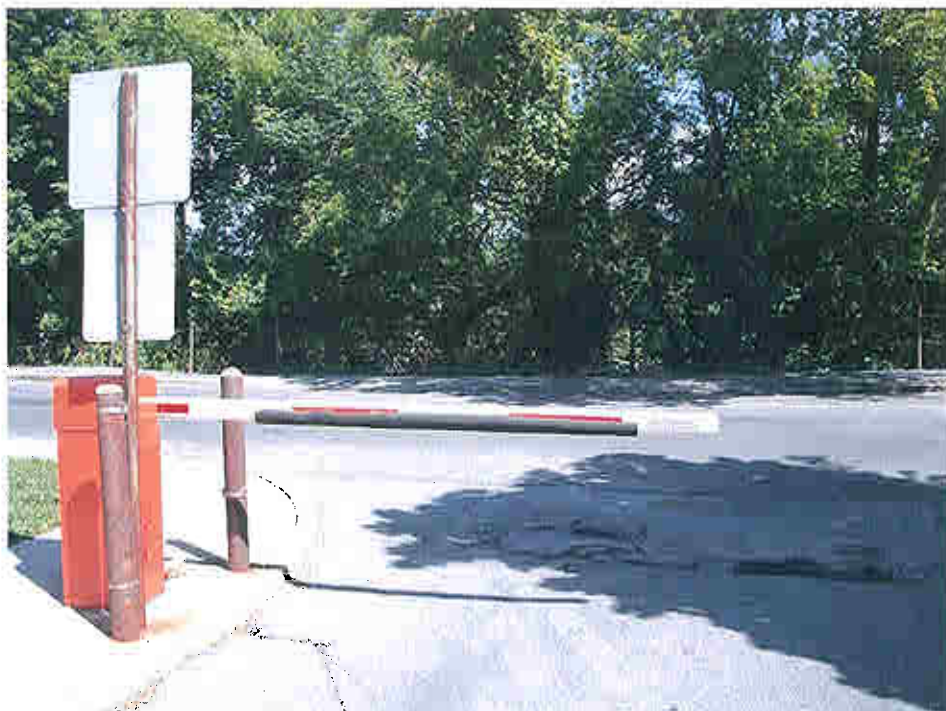
Photo 7 - Precipitation sheet flows from the Parking Lot thru the Exit, across University Avenue, over the drop curb, over the asphalt sidewalk, over the retaining structure, into the gorge.
