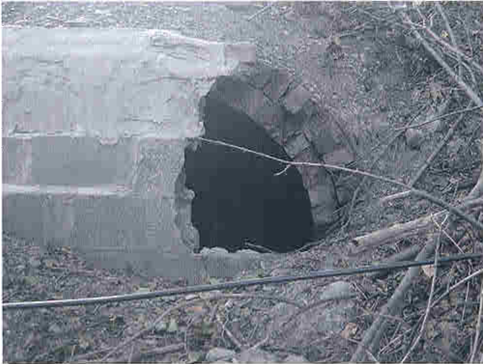
Photo 19 - Tunnel under University Avenue.
