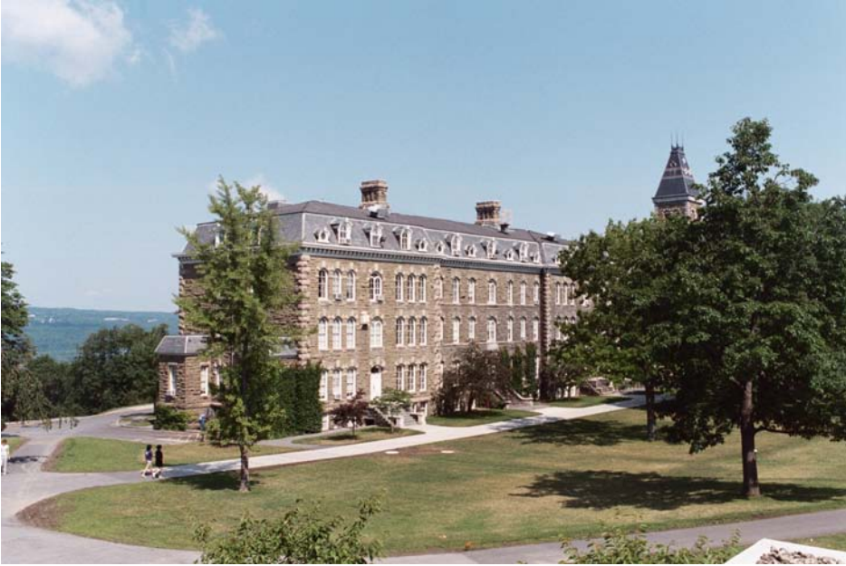
Figure 38 Morrill Hall – south and east facades, view from south end of Arts Quad
