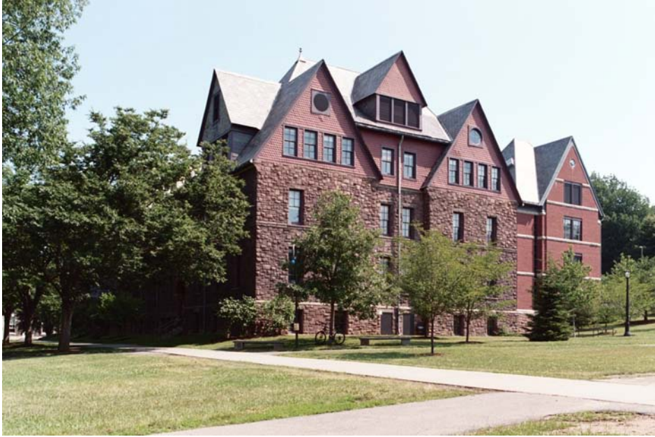
Figure 32 Lincoln Hall, from Arts Quad - south façade. 2000 addition at right
