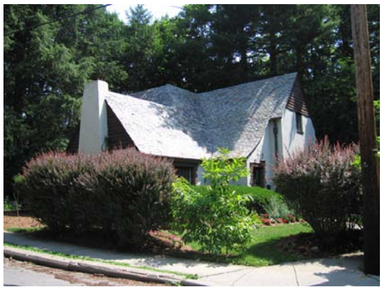
302 Fall Creek Drive (north side)
