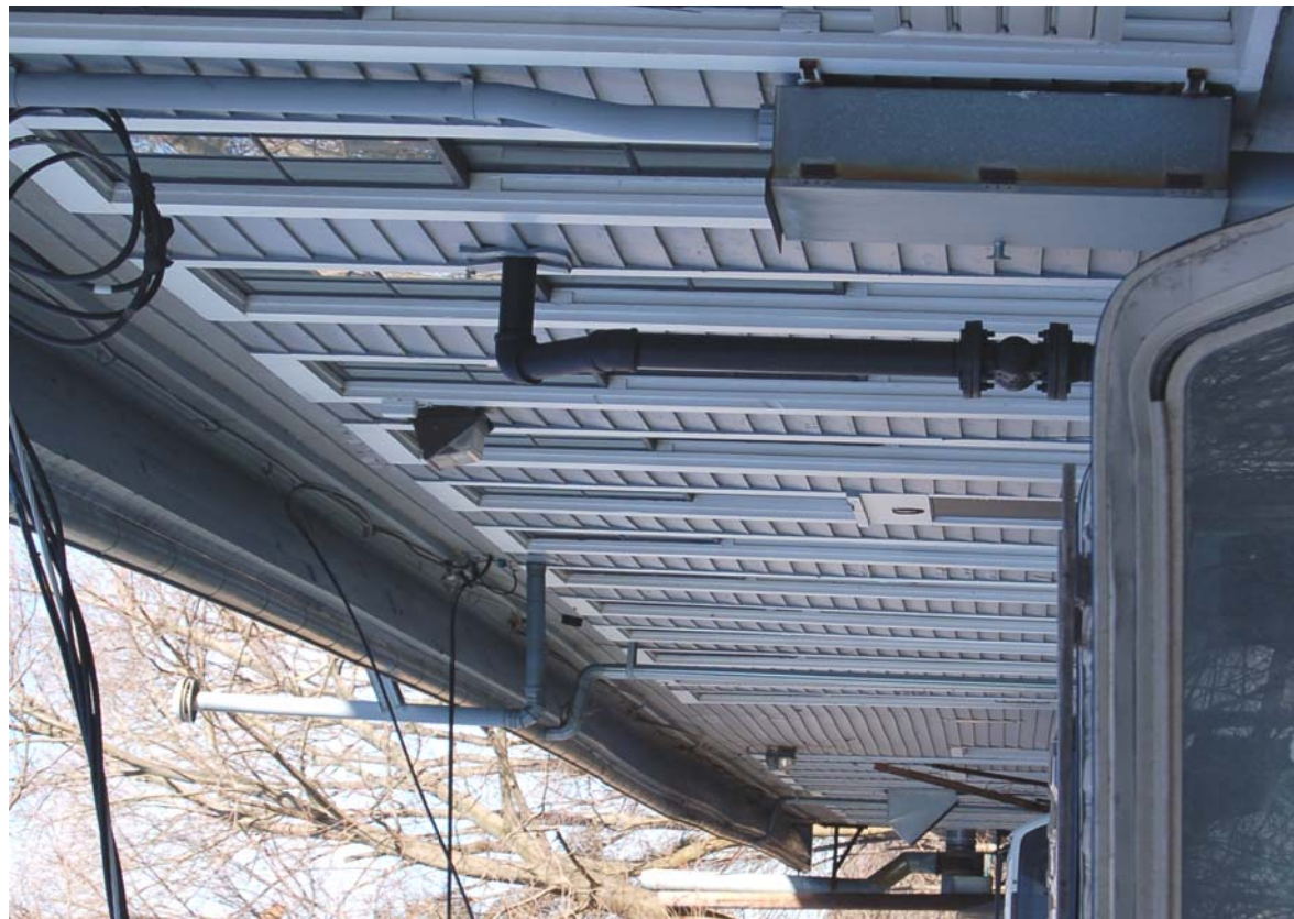
WALL MOUNTED FIXTURES ON THE NORTH FOUNDRY FACADE
