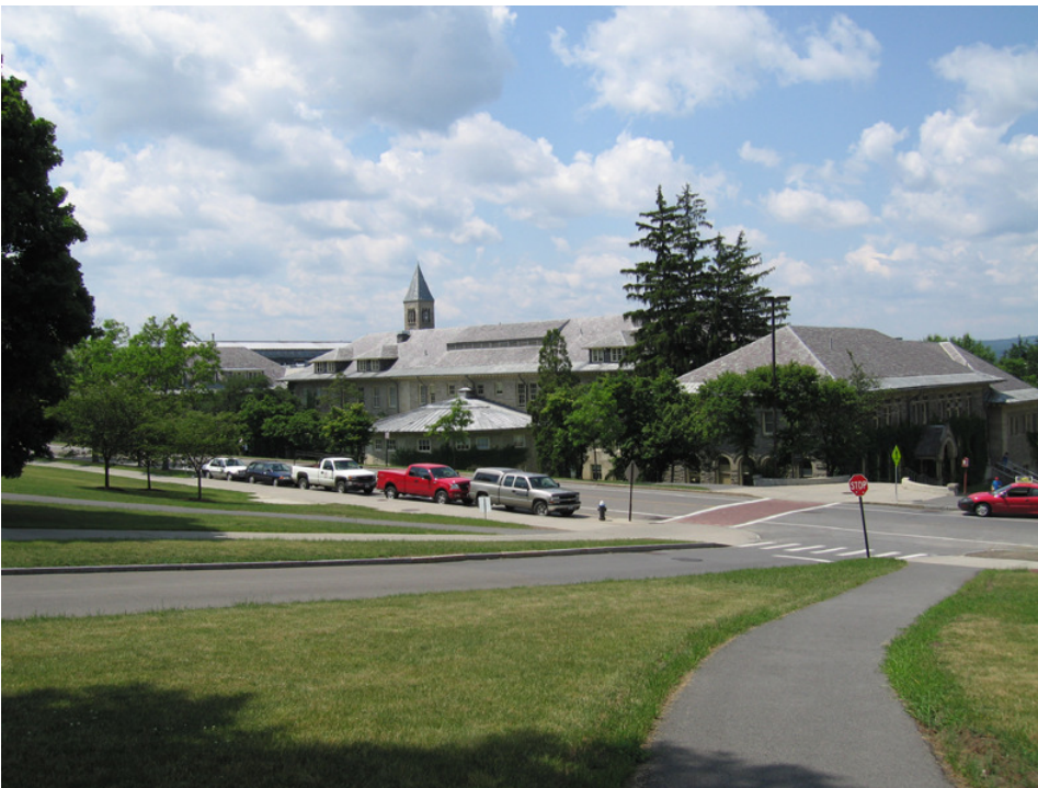
Figure 34 Goldwin Smith Hall from east. North section ( right ) is former Dairy Building
