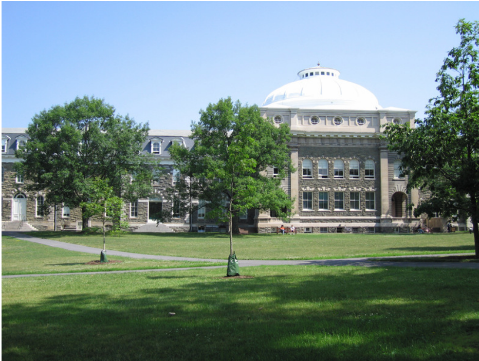
Figure 25 West Sibley Hall and Sibley Dome, from south
