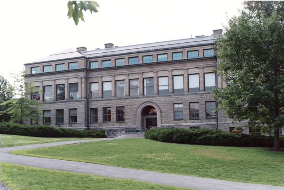
Figure 35 Stimson Hall, north facade
